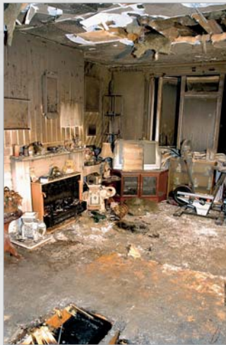
The devastating consequences of not having a smoke alarm installed.
